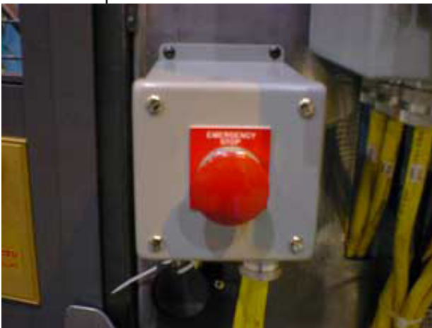
Photo 2 – This more modern button is non-compliant due to the RED background and spring-return button.
