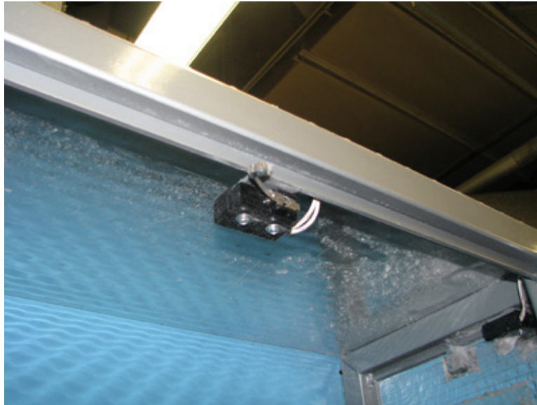
Photo 1 – Micro-Switch style limit switch used as a cover interlock switch in a piece of industrial laundry equipment
